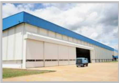
External side view of the hangar
