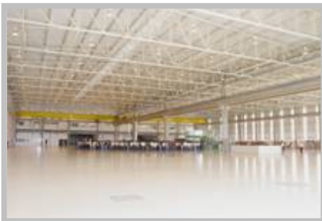
Final assembly area at new hangar in Gavião Peixoto
