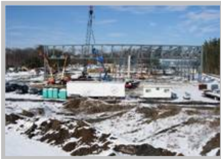
Service Center at Bradley Airport, Connecticut
